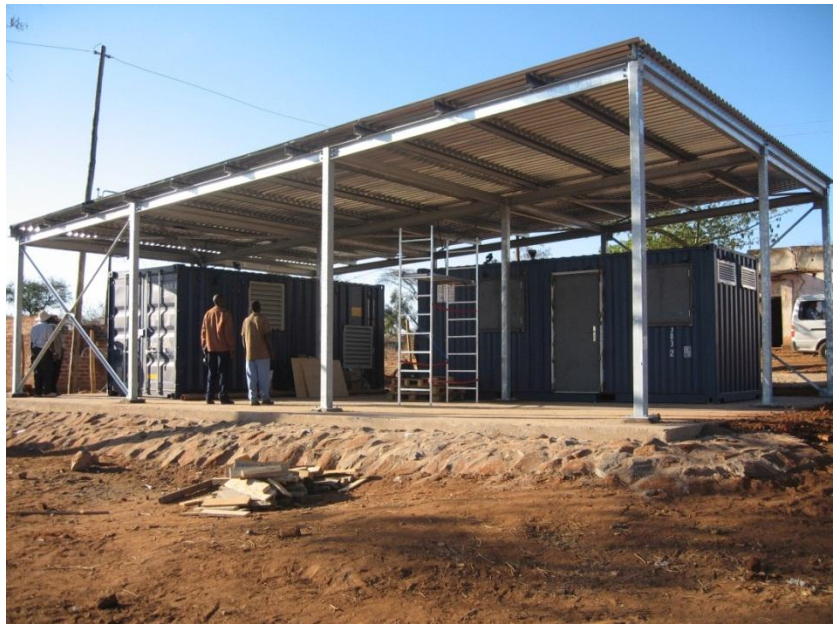
Figure 2 The finalised 13.5 kWp installation, in which the two shipping containers were utilised to house the system switch gear and the other as an office for the project established village cooperative.
